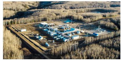
Our Septimus natural gas plant uses hydroelectricity to run the electric compressor motors
