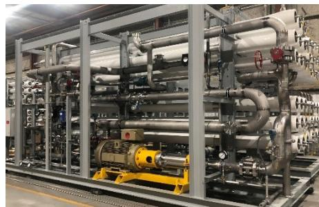
Reverse osmosis treatment system at PAW improves water recycling capabilities and reduces natural gas consumption
