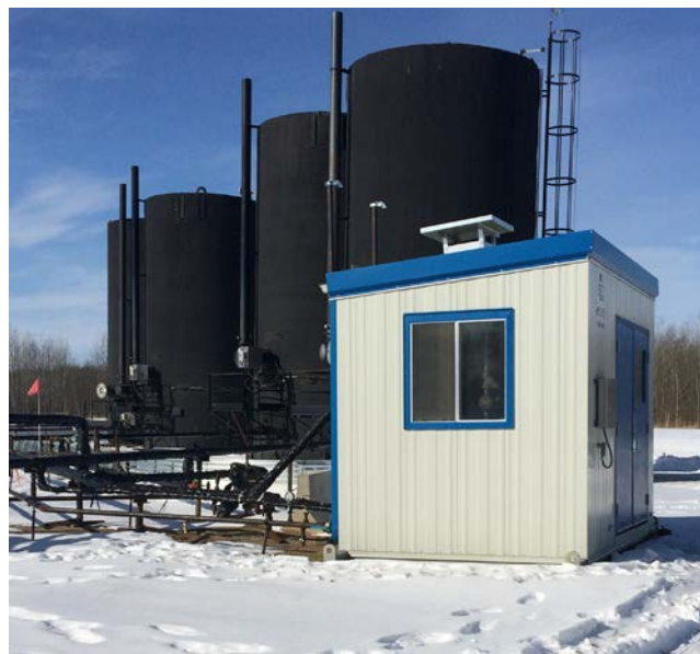
Solution gas conservation compressor unit at Bonnyville facilities.
