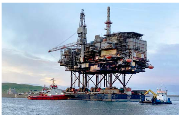
Ninian North Platform topsides being transported to the quay (platform for loading/unloading vessels).
