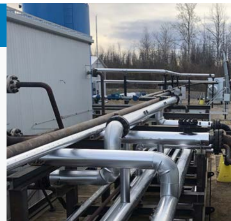
Natural gas re-injection piping at LEGS pilot.
