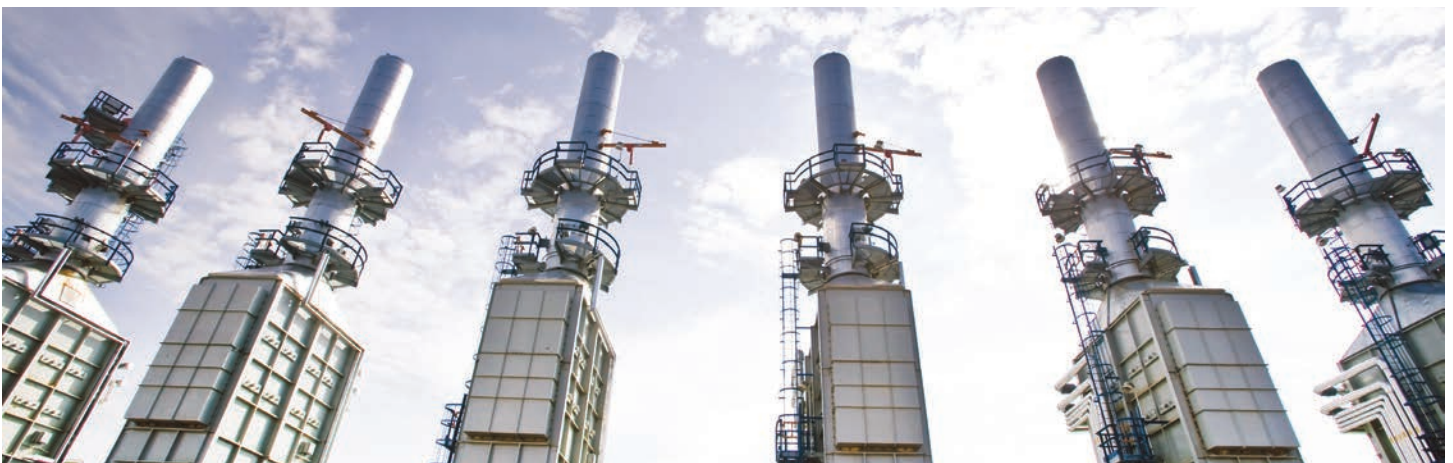
Steam generators at Jackfish thermal in situ facilities.
