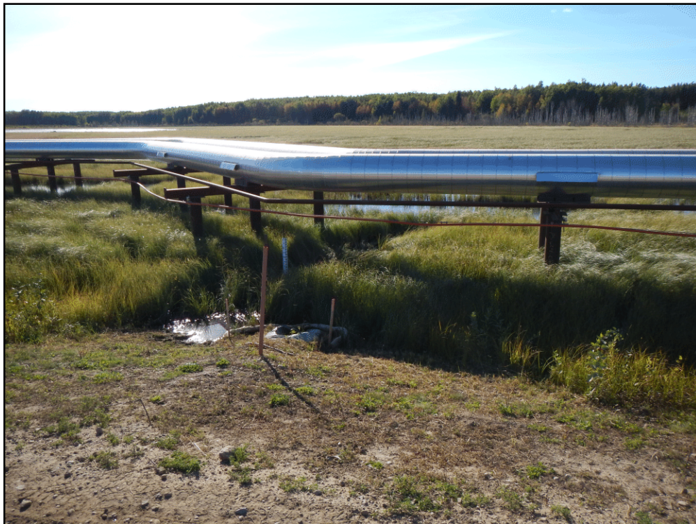
2. Facing southwest toward Basin 3 - September 19, 2013.
