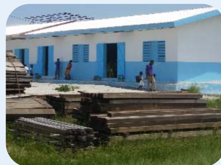
New classroom built by Canadian Natural
